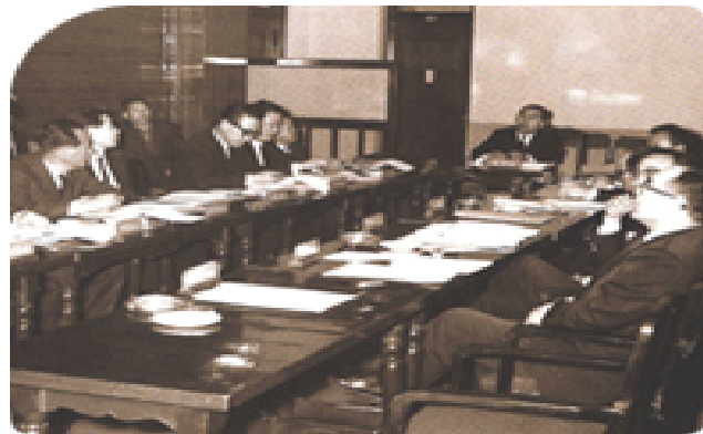
Integrated Steelworks Construction Project Promotion Committee meeting
