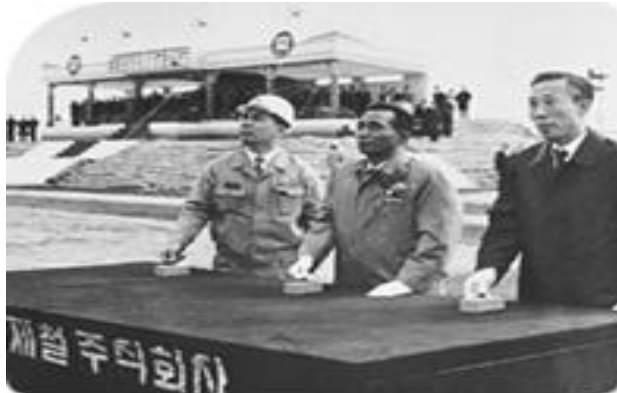
Construction of Pohang Works Phase 1 begun
